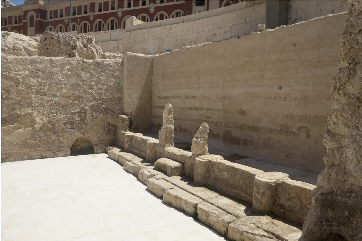
Fig. 6. The southern wall of the court of Hypogeum A in Shatby, constructed with blocks cut from the mother rock. © The Archaeological Society of Alexandria.
